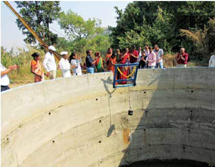
Well construction - Rural development project
